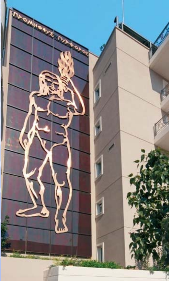
Experimental office building ReSEL/ENVTUC
