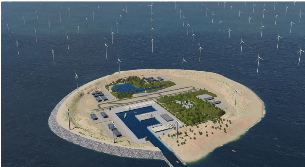
Figure 10 Design for artificial island hub in the North sea. It will be equipped by solar panels and 7000 wind turbines. Source: TenneT
